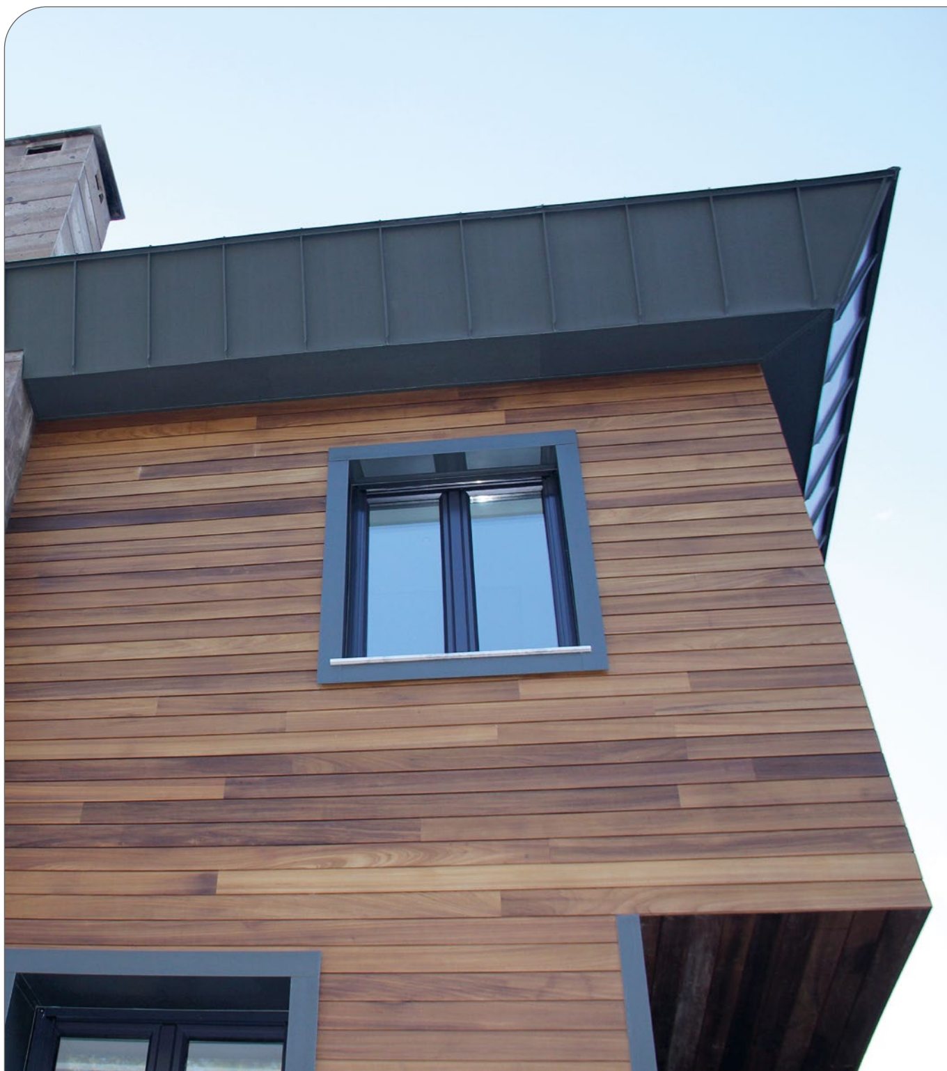
Figure 46. ThermoWood® exterior wall cladding.
