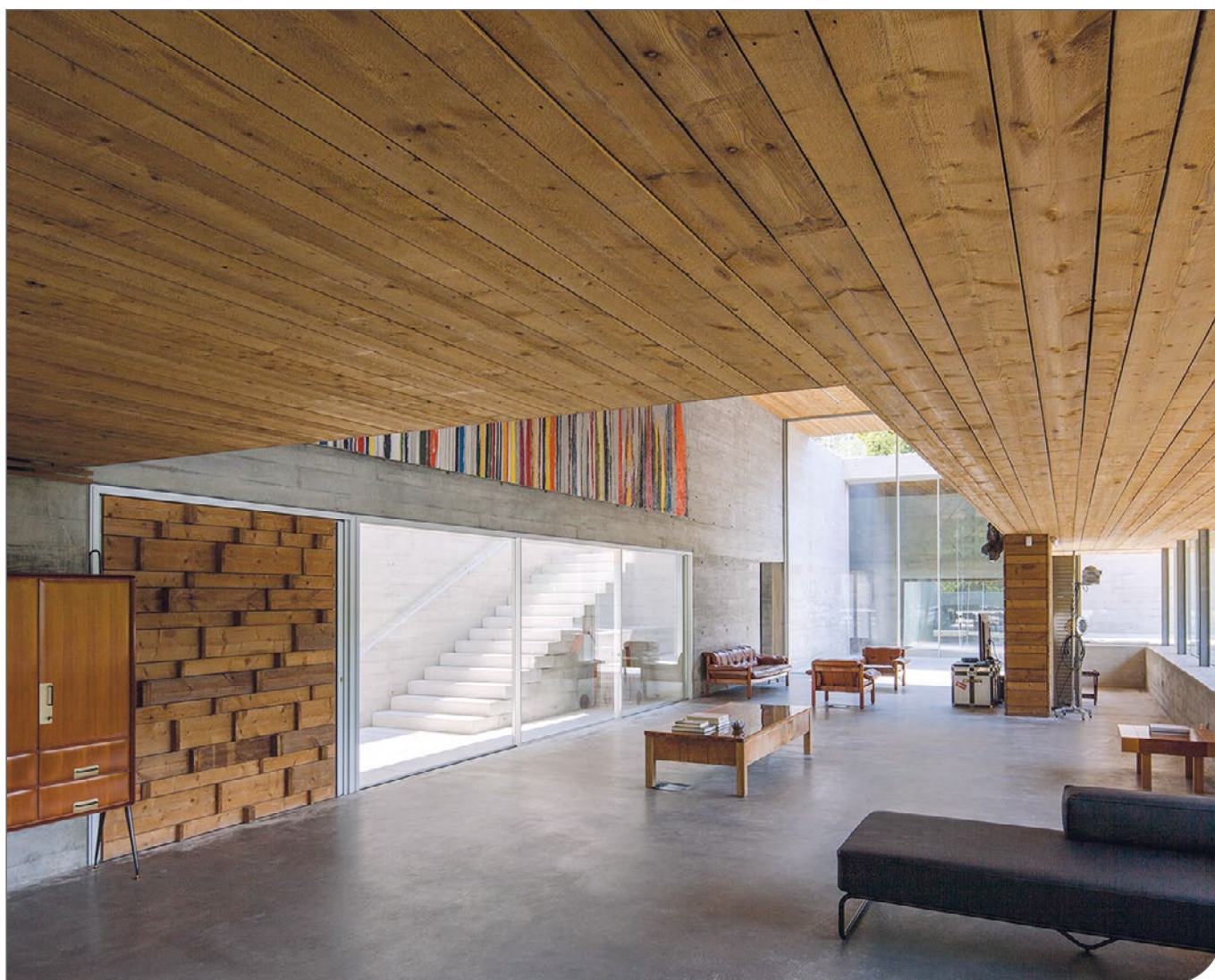
Figure 37. ThermoWood® ceiling in Portugal
