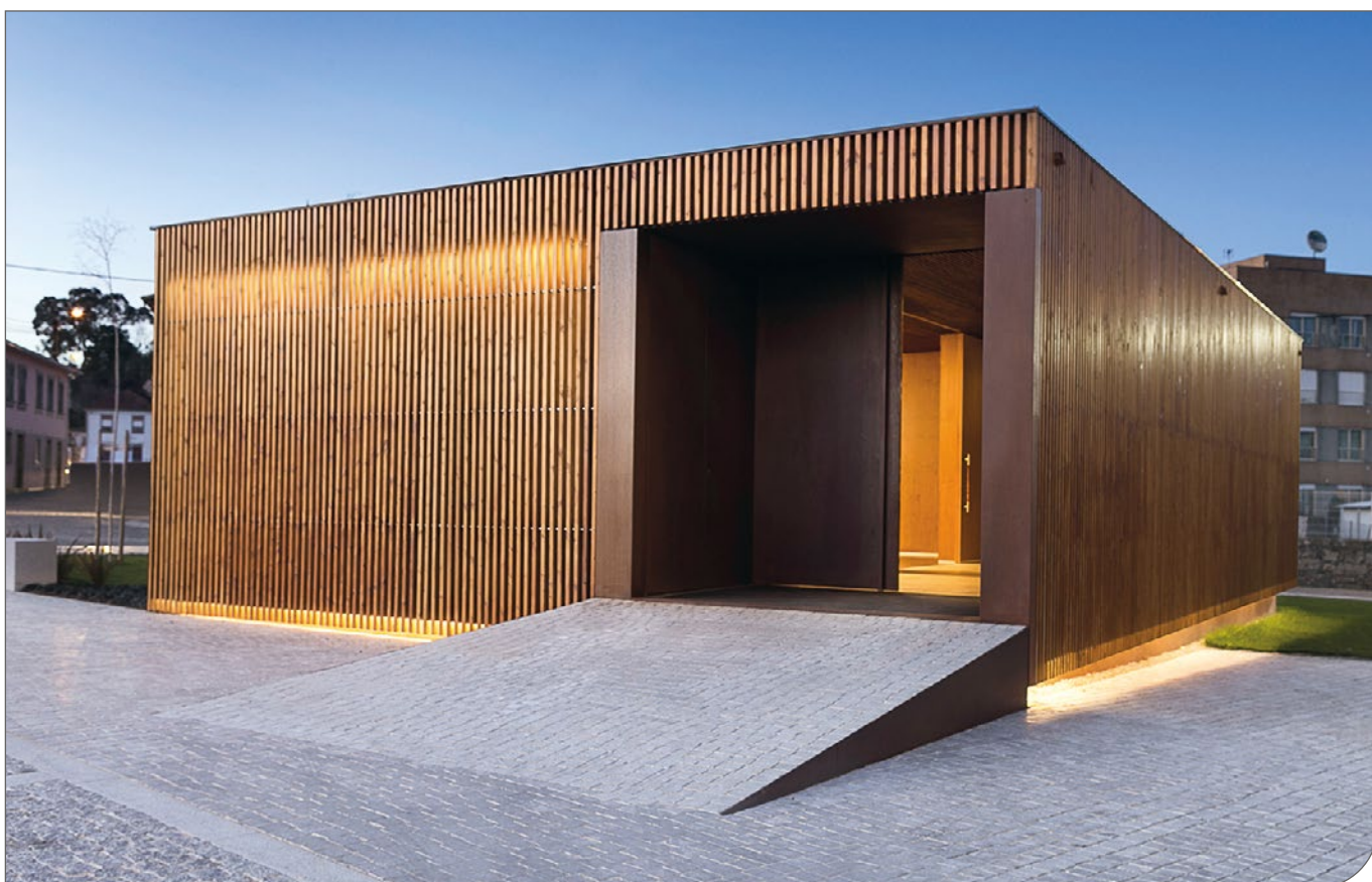
Figure 68. ThermoWood® exterior wall cladding on a Portuguese church.
