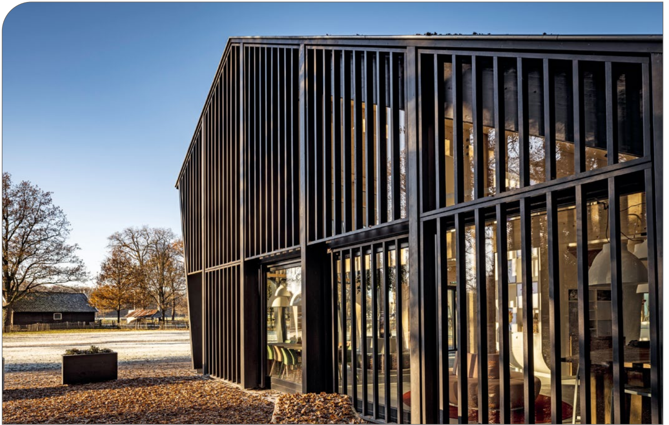
Figure 69. ThermoWood® exterior cladding (Netherlands).
