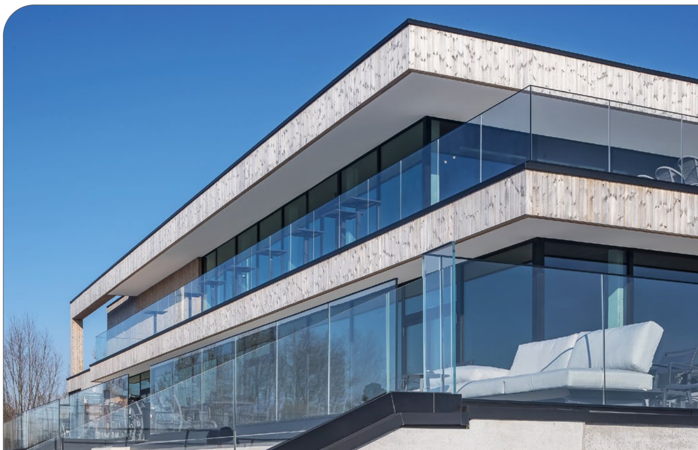
Figure 71. ThermoWood® exterior cladding (Belgium).
